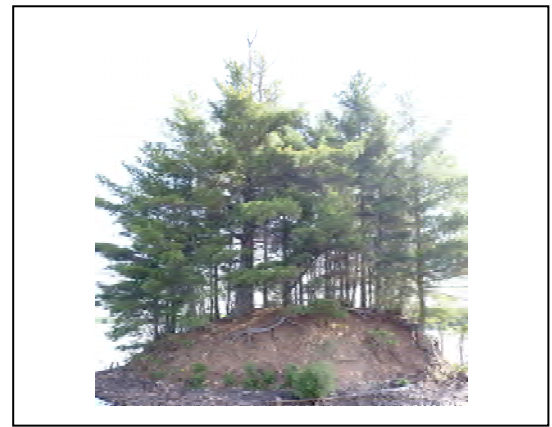
40. Island #8 – Bank erosion
