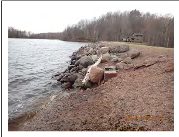
37. Gile Dam Canoe Portage – Riprap shoreline of flowage, west of dam
