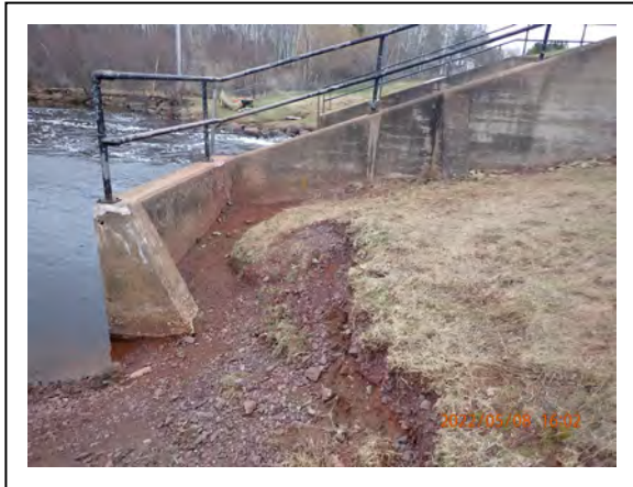
31. Gile Dam Canoe Portage – East side of Intake
