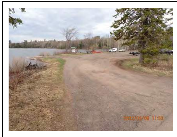
80. County Hwy. C Landing – Entrance and Parking
