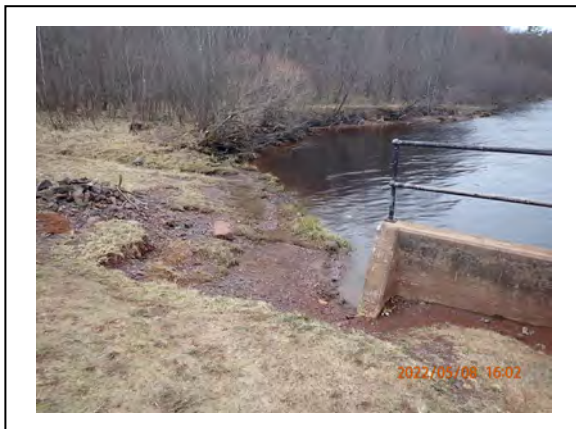
33. Gile Dam Canoe Portage – Left Descending bank of Tailrace (1)
