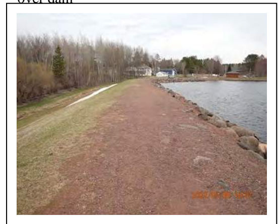
42. Gile Dam Canoe Portage – East side of dam, riprap shoreline of flowage
