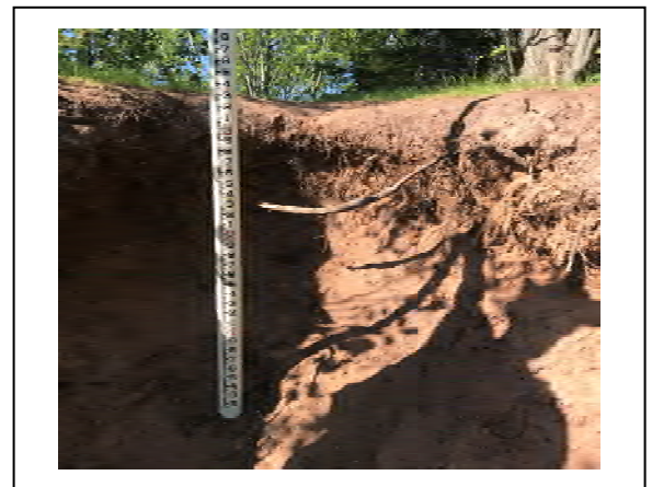
154. Island #35 – Bank erosion
