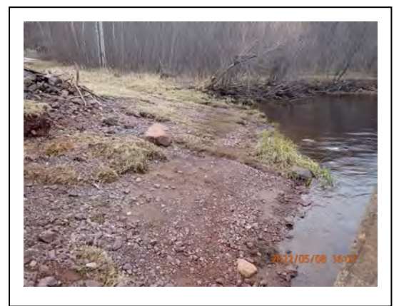
34. Gile Dam Canoe Portage – Left Descending bank of Tailrace (2)
