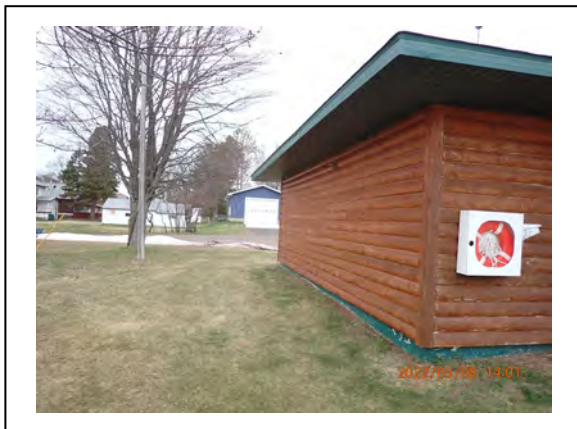
21. Gile Park – Restrooms (2)
