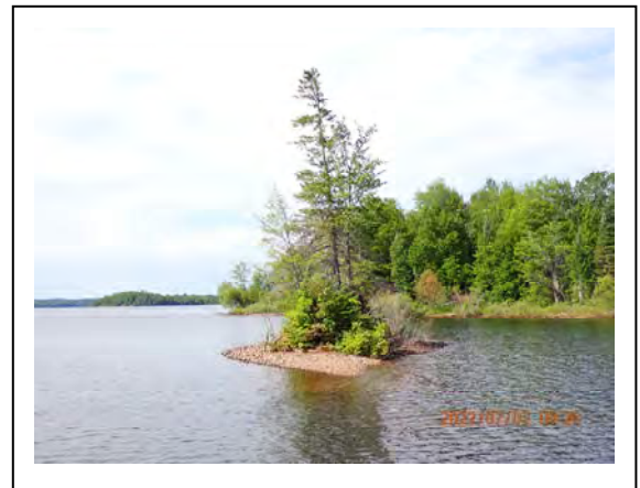
38. Island #7 – Shore erosion
