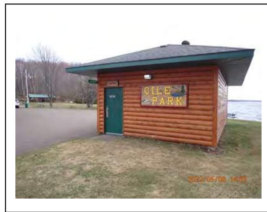
22. Gile Park – Restrooms (3)
