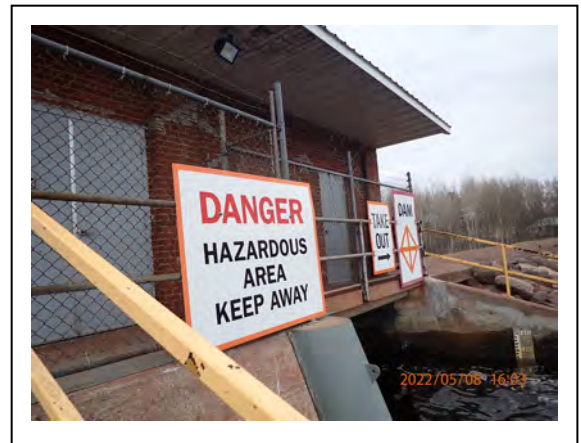
38. Gile Dam Canoe Portage – Intake signage
